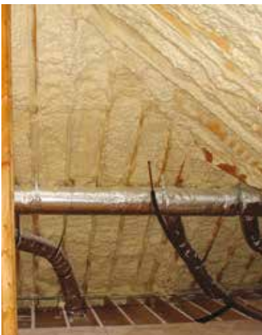
Attic with spray foam insulation
