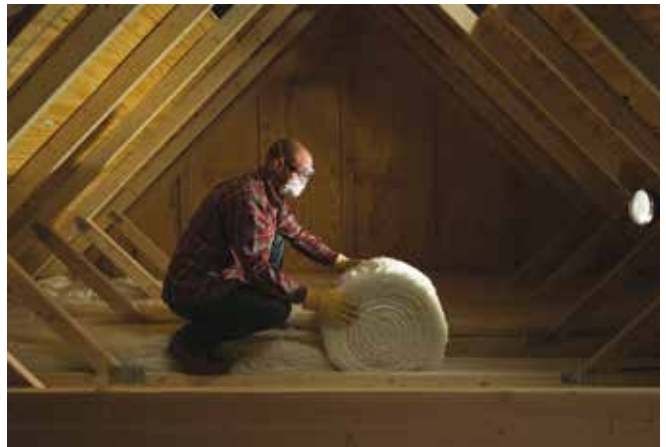
Rolling out batts of insulation
